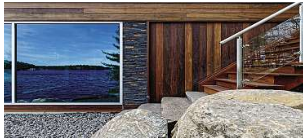
The large window walls facing the lake are completely non-structural.
